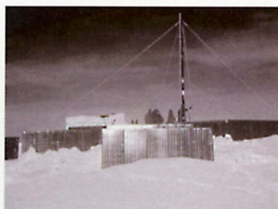
An array of 60 photovoltaic cells used on the col of Huascarán in 1993 produced four kilowatts of power.
