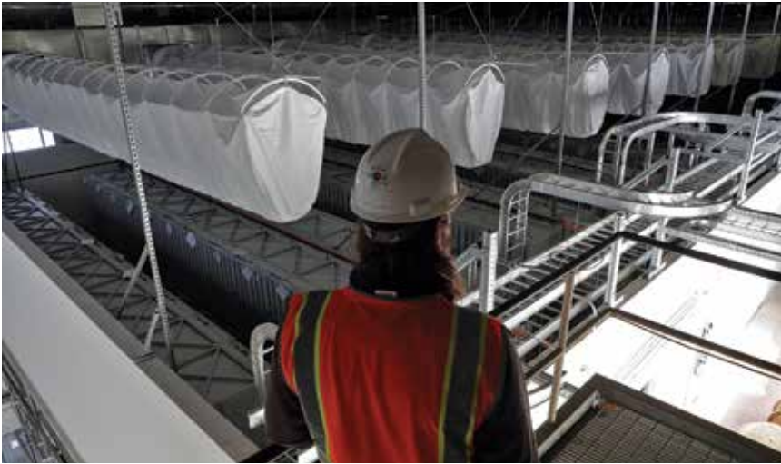
David Yeager, project manager for Vistra Zero, looks over the battery array in the old generator building at the Moss Landing Power Plant in Moss Landing, Calif., on January 13, 2021. Vistra Zero is the largest energy storage system of its kind in the world, able to store up to 300Mw of power. It uses lithium-ion batteries to capture excess electricity from the grid and release it when needed later, typically during solar and wind down times. CARLOS AVILA GONZALEZ/THE SAN FRANCISCO CHRONICLE/GETTY IMAGES
